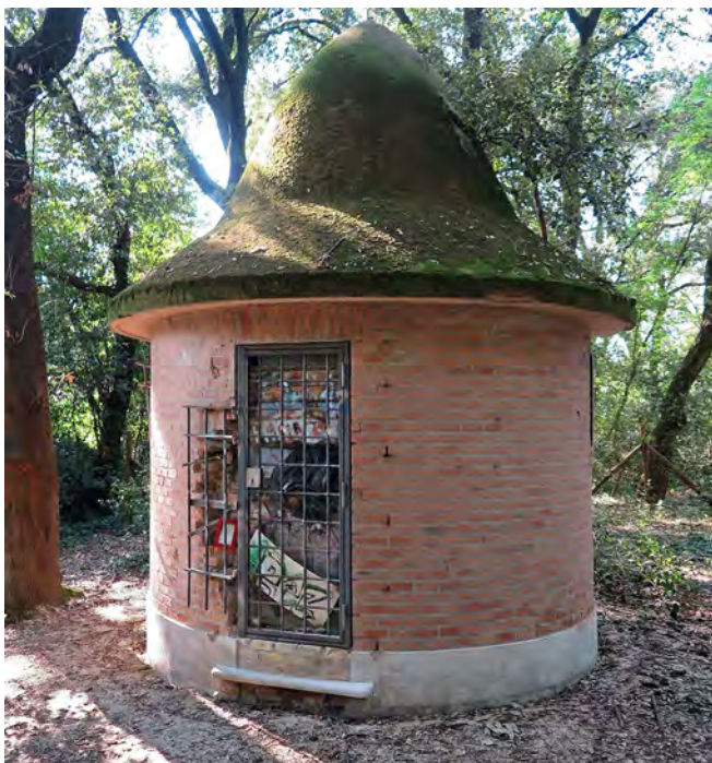
The distinctive emergency exit atop the Villa Ada shelter
